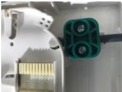
Cable Clamp in JW2 Box
